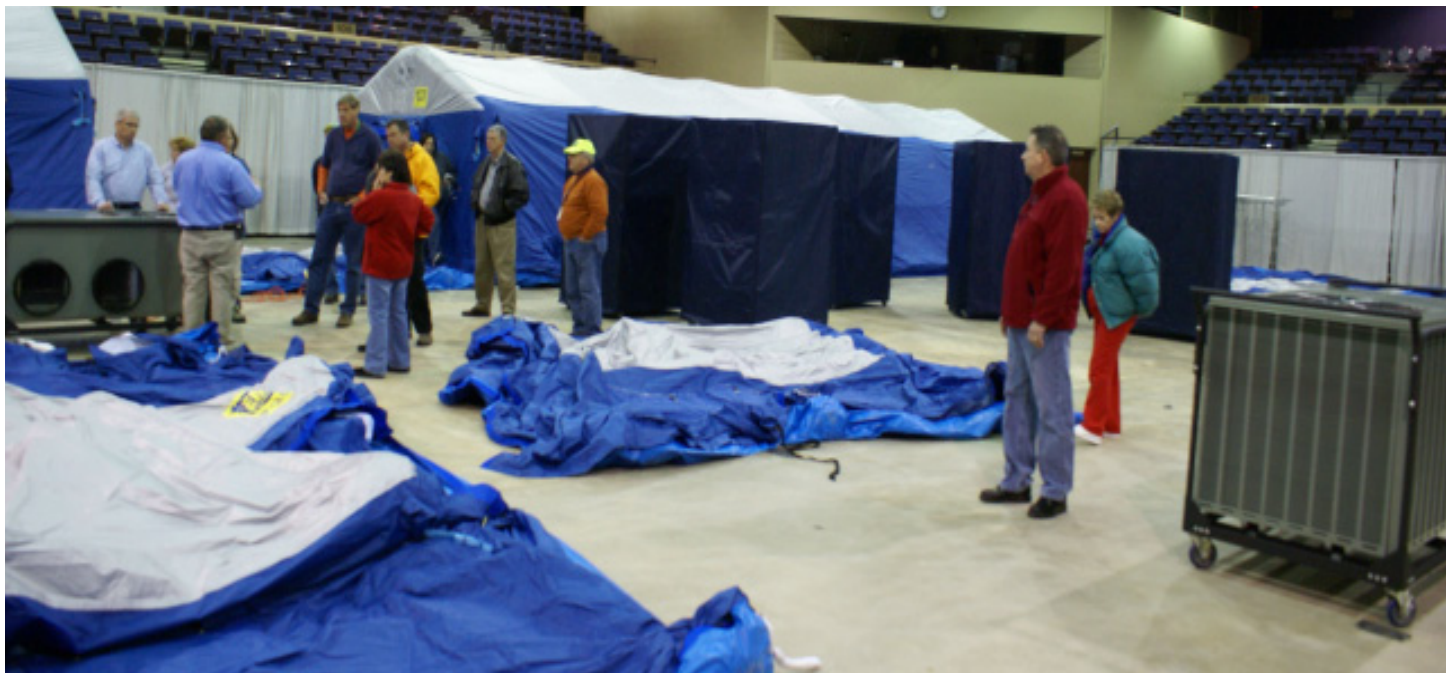
Bottom: Volunteers listen for more instructions on how to position the hospital rooms. The bed racks (dark blue units), air conditioning units, and additional hospital rooms have been unloaded and prepositioned for installation.
