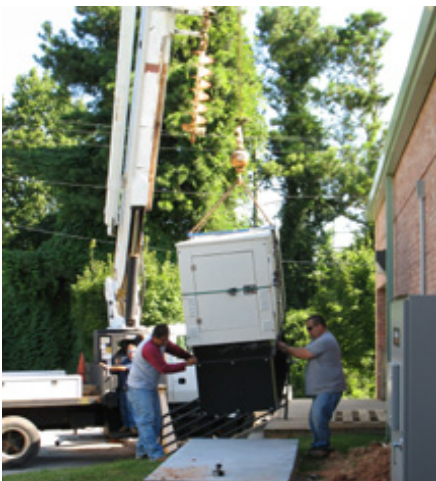
Top right: unloading the generator
