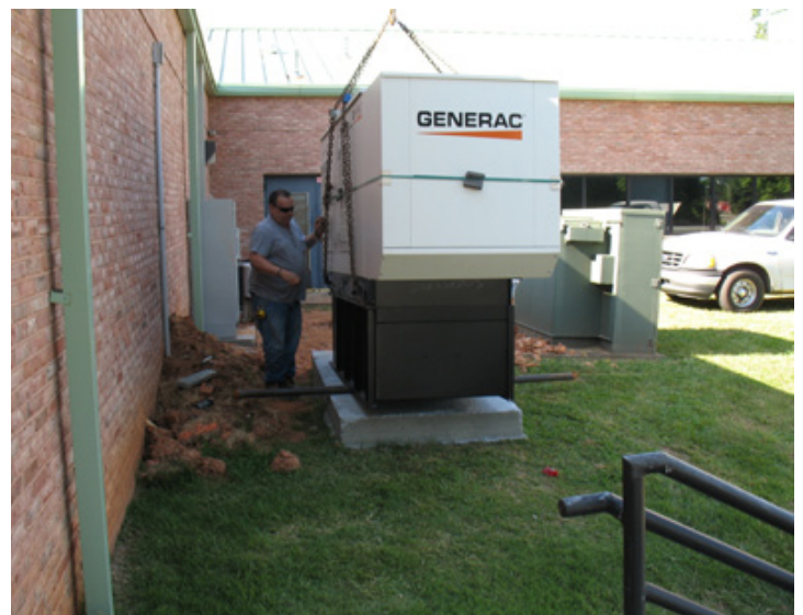
Right: ready to install the generator
